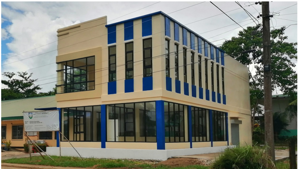
■ Construction of a new library building at CapSU Pontevedra
