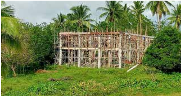
On - going Rehabilitation/Expansion of Poultry at CAPSU Burias
