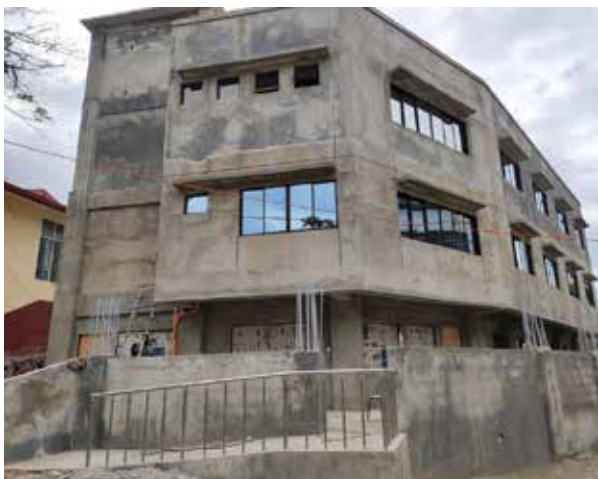
■ Ongoing Construction of three-story multi-use building (Roxas City)
