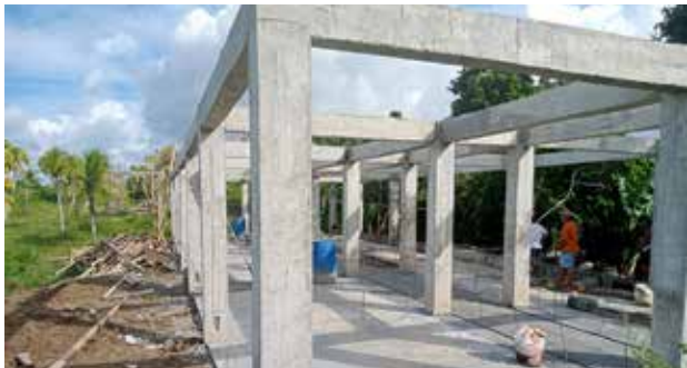
On-going Rehabilitation/expansion of Growing Area (Piggery) at CAPSU Burias
