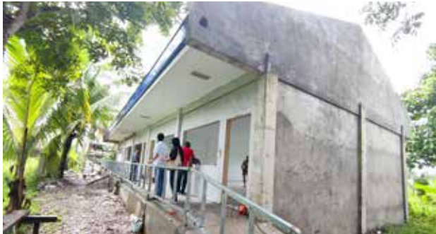
On-going Reconstruction/ Rehabilitation of Industrial Technology Building at CAPSU Sigma
