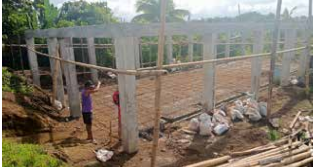
On-going Rehabilitation/Expansion of Piggery (Breeding Area) at CAPSU Burias
