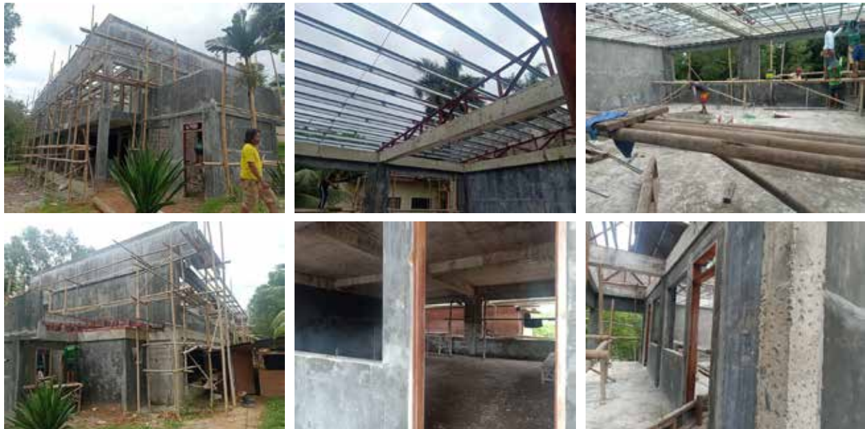
On-going Renovation/Expansion of Veterinary Medicine Academic Building at CAPSU Dumarao
