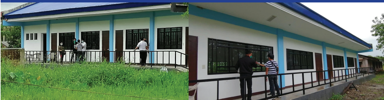
RECONSTRUCTION / REHABILITATION OF THE INDUSTRIAL TECHNOLOGY BUILDING AT CAPSU SIGMA
