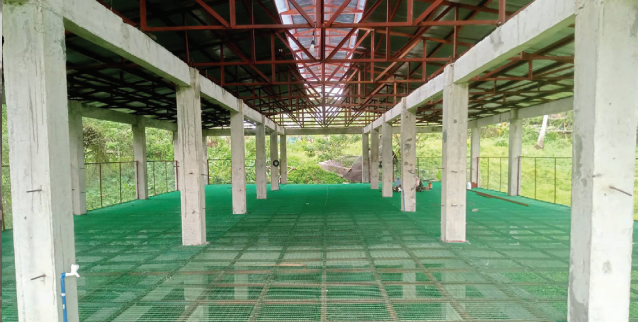
The structure ready for stocking
