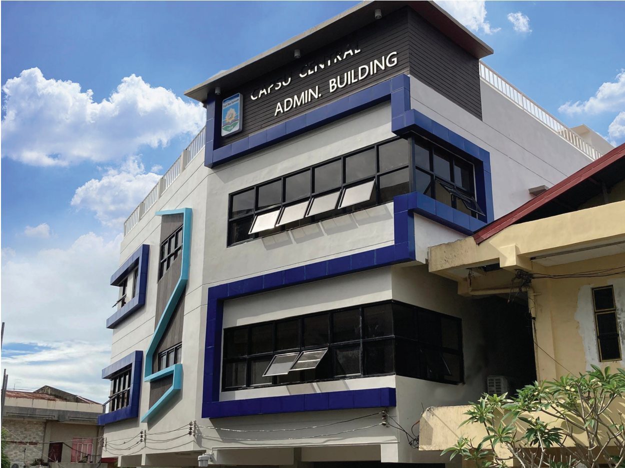
The completed expansion of the Central Administration building that house the offices of the University President, the VP Admin and Finance, the Accounting dept, the Cashiering, Internal Audit, Budget, CAO (Finance and Administration), Board Secretary, HR, and Records.
